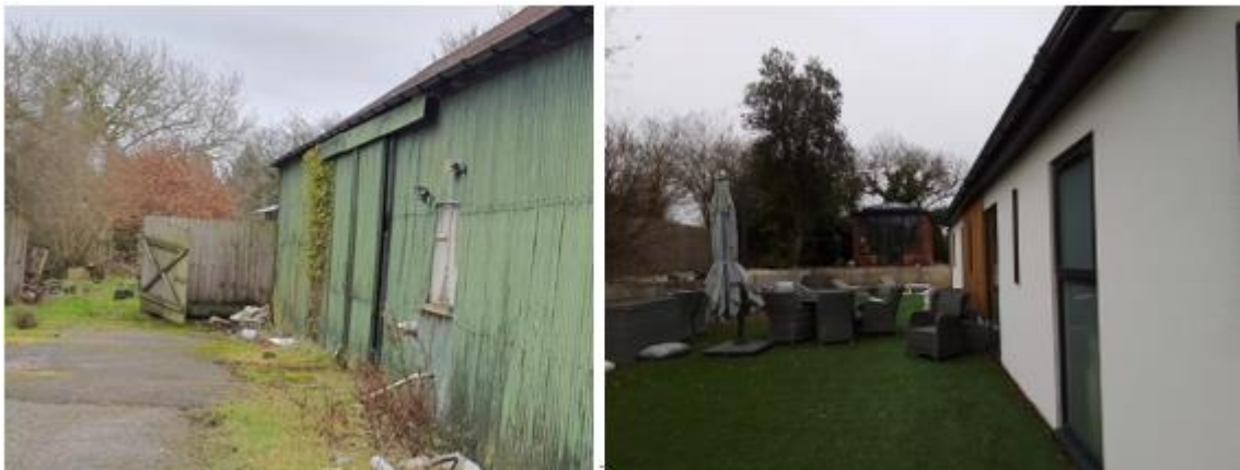
Figure 3 – Photograph above left (submitted by agent on 19/01/2021 for application 3/20/2281/PNAGD above left, and the Photograph to the right taken during officer site visit on 12/12/2024 (above right)
